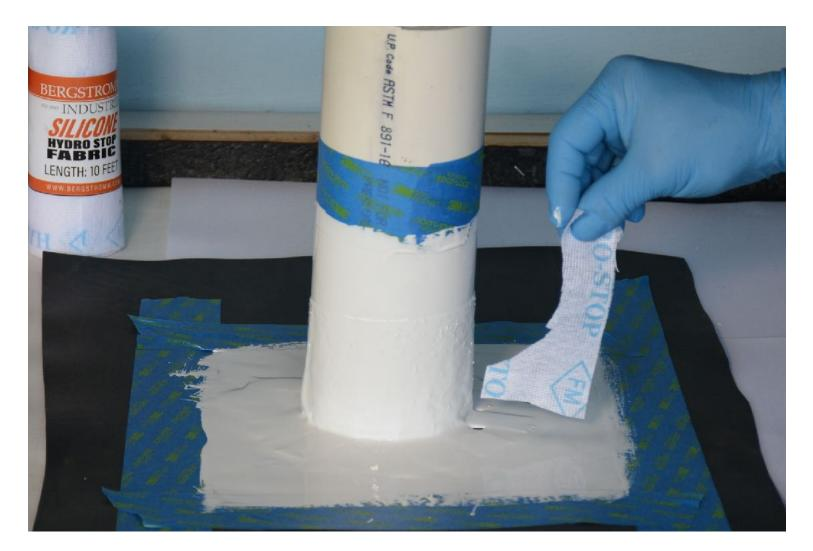
• Paint a thick coat so you can't see the texture of the fleece. Put a small piece over holes
