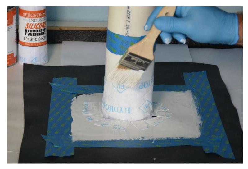
• When installing the fleece, make sure the tabs are lying flat.
