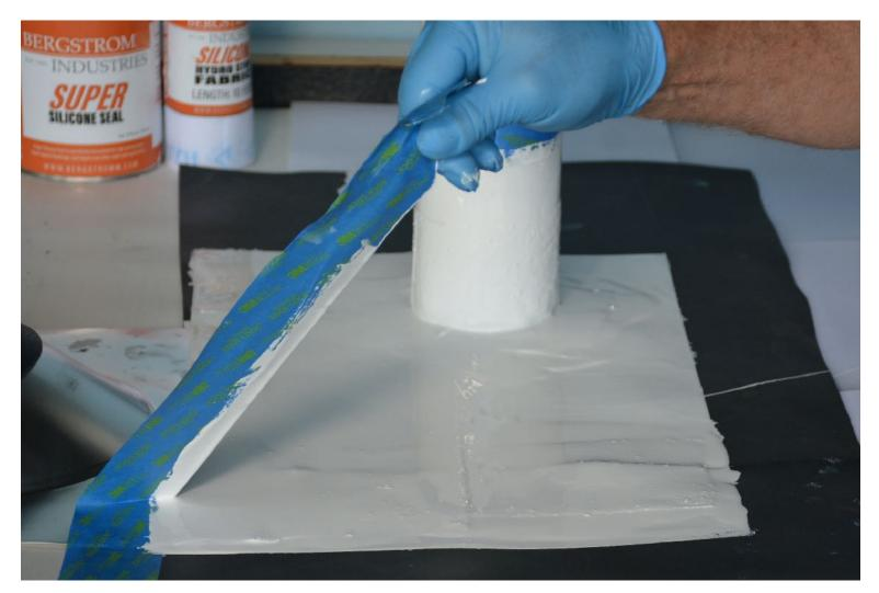
• Remove the masking tape immediately after applying the last coat
