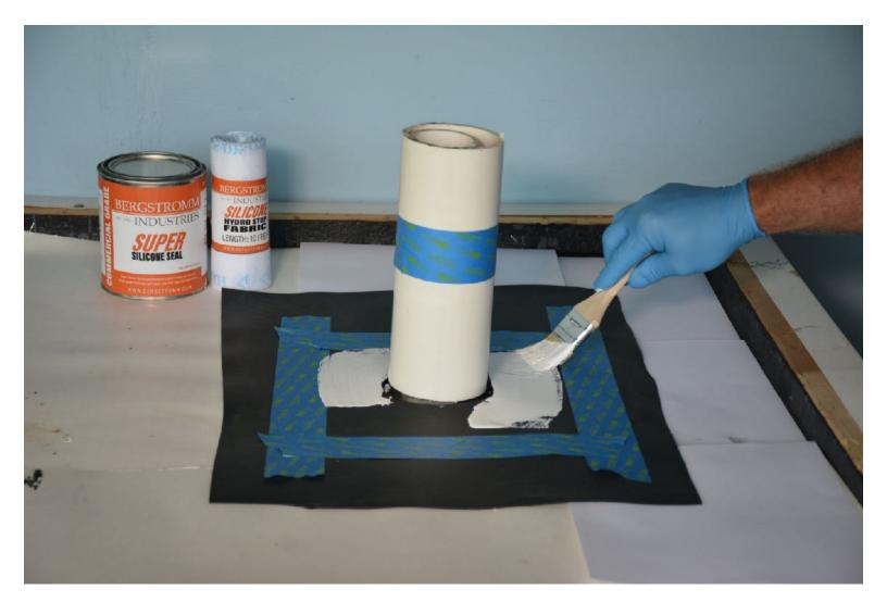
• Apply a thick coat of Super Silicone Seal to both surfaces - pipe and roofing surface
